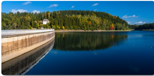
Saidenbach drinking water reservoir, Germany
